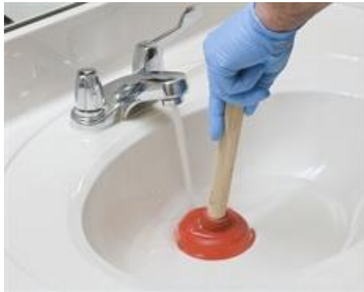
Sinks or toilets backing up or draining slowly, in spite of using plungers and drain cleaner
