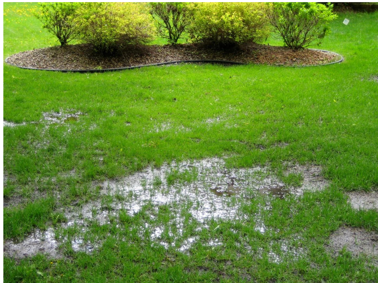
Wet areas, lush grass, or foul odors around the drain field.
